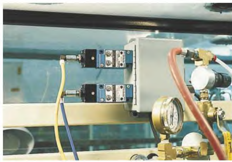
Figure 13-17 Pressure to current sensor for low pressures.
