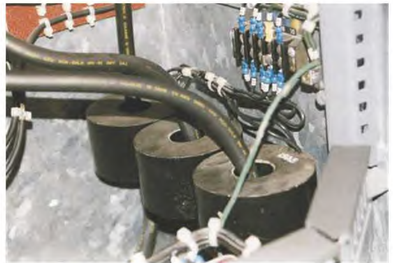
Figure 4-31 Current transformers reduce overload current.
